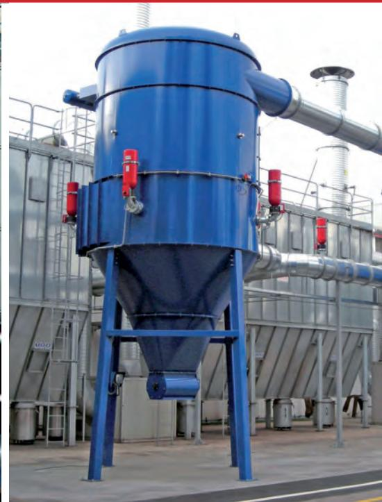
Dry filtration: sleeves pockets, cartridges
